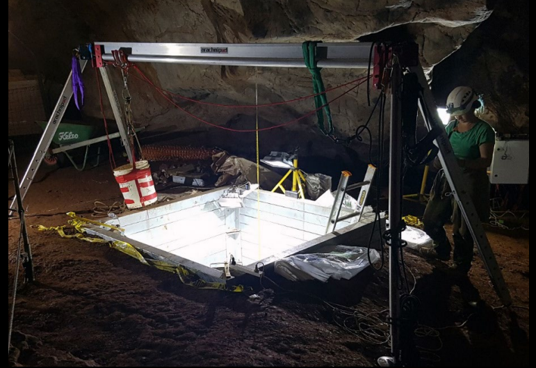
Excavation pit after shoring
