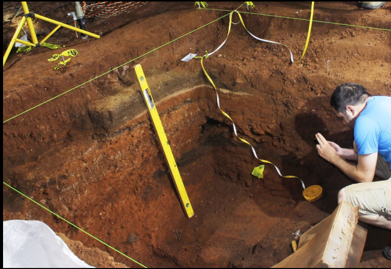
Excavation pit before shoring
